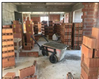
Fig 3: Masonry design at a construction site - service optimization – [8]. Source: the authors.
