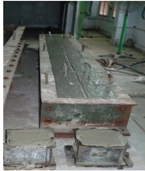
Fig 4: Casting of geopolymer concrete
