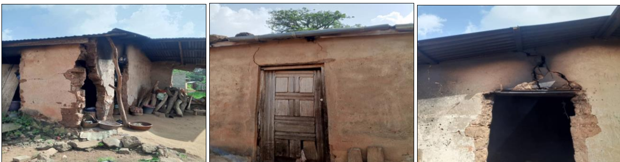
These photos show the impact of vibrations caused by regular mining operations on the stability of habitats in the village of Oualéguéra.
