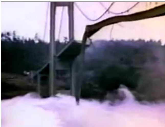
Fig 1: Tacoma Narrows Bridge Collapse
