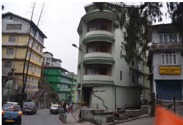
Fig 3: Several structural cracks identified 6 multi stored building
