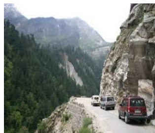
Road in Kiza
